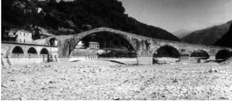
The paper reports on a vibration measurements campaign performed on the medieval Maddalena Bridge, also known as the "Devil's Bridge", in Borgo a Mozzano (Italy), one of the most fascinating in Italy. This 11th century masonry bridge, supported by four circular arcades, crosses the Serchio River
